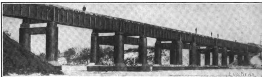
FIG. 8. OXFORD MILL POND BRIDGE; CHICAGO & NORTHWESTERN RY. (When the dam is raised the water level will be just below the plate-girder struts connecting the tops of the piers)
