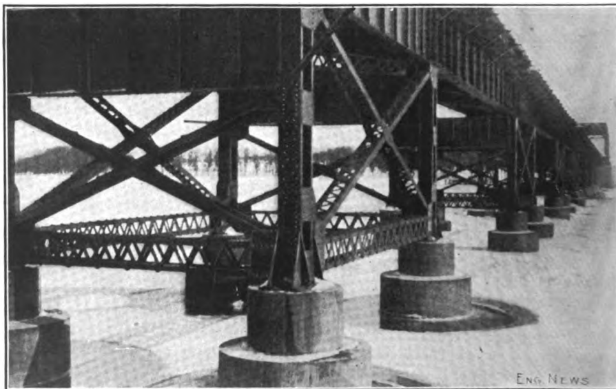
FIG. 5. BUFFALO LAKE BRIDGE, SHOWING STEEL SUPERSTRUCTURE ON CYLINDER PIERS (JANUARY, 1912); CHICAGO & NORTHWESTERN RY.
